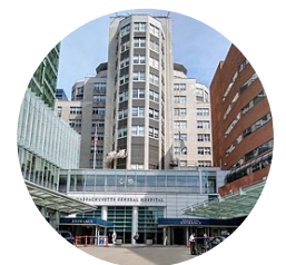
Massachusetts General Hospital (Boston, MA)
